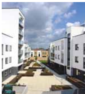
82 new homes just completed Watermark, Waltham Forest
