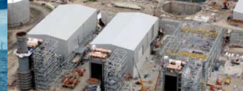
Gas-fired CHP construction at Grain
