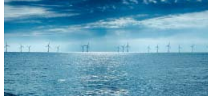
Offshore wind farm
