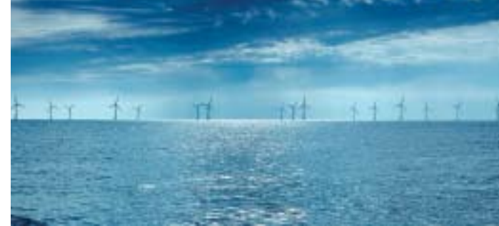
Offshore wind farm
