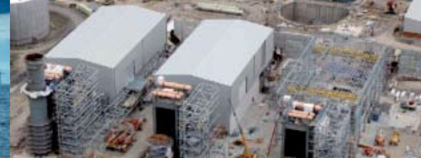
Gas-fired CHP construction at Grain
