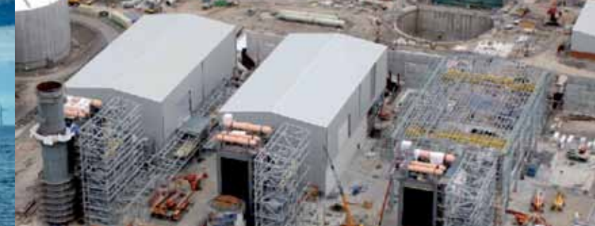
Gas-fired CHP construction at Grain
