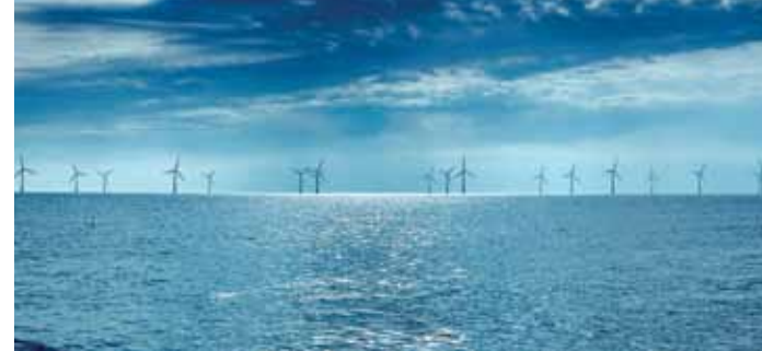
Offshore wind farm
