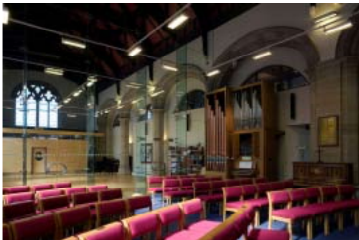
View to the West end of the Church showing the new full height glazed screen and new kitchen and toilet accommodation.
