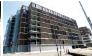
596 space public car park
